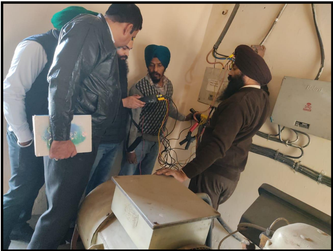
Energy audit going on
