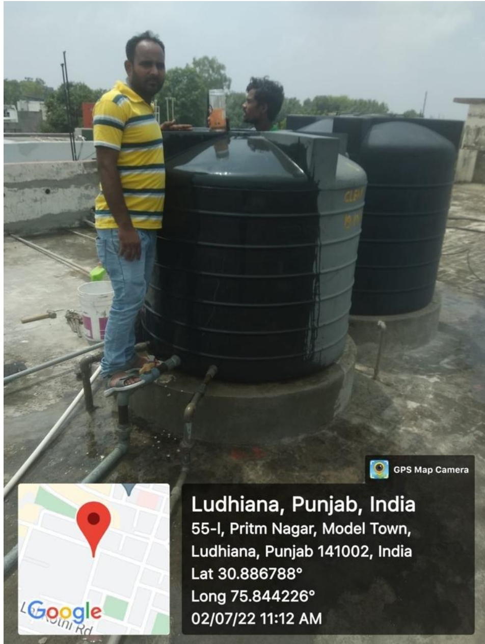
Cleaning of water tanks
