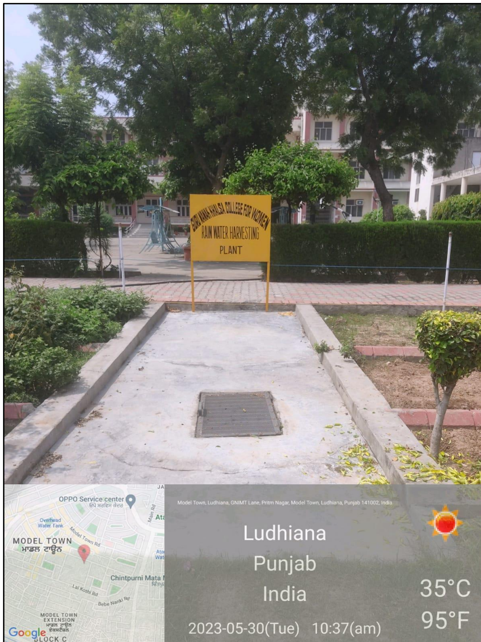
Rain harvesting system available at college campus
