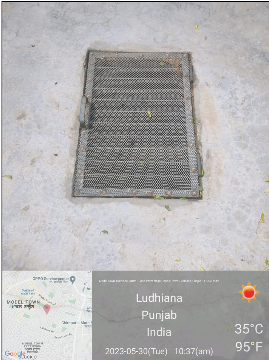
Rain harvesting pit
