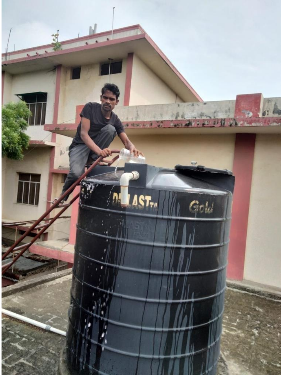
Cleaning of water tanks
